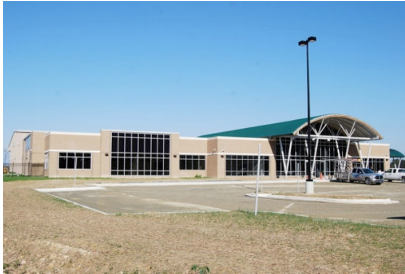
Roanoke Electric Coop's main facility in Ahoskie, NC where wireless video surveillance systems are implemented.
